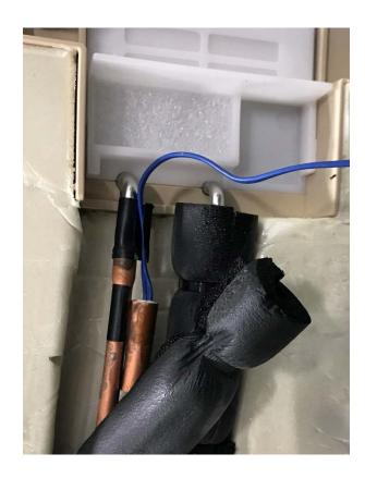
4. The blue wire shown above terminates at the Cold Temp Sensor. Cut away the black electrical tape and remove the sensor. If replacing, trace the wire back to the PCB and unplug from the board. When placing the new sensor, wrap with electrical tape to secure it in the tubing sleeve and return all foam pieces to original position.
