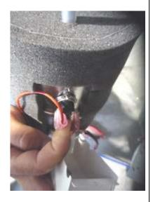
7. Reattach the Protective Metal Box by depressing the top flap of the Protective Metal Box so it snaps back into its original position on the hot tank.
