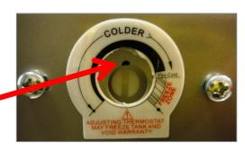
Turning the adjustment screw clockwise to lower the set point temperature.
