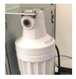
3. After adapting to the cold-water side of the water source, insert 3/8" tubing into the "IN" port of the filter head. Assuming the filter has already been flushed, run 3/8" tubing from the "OUT" port of the head to the bulkhead on the ice machine. Turn water "ON" and check for leaks. **NOTE**: Max water pressure is 60psi.
