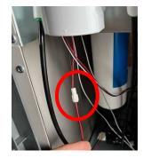
5. **Flush the prefilters**. Disconnect the tube connected to the left side of the first filter head (circled in RED). Using a ¼" union, add a length of tubing to reach the drain or a 5-gallon bucket to the end of the tubing removed. **Plug the unit into power**. Turn the water supply ON and allow 2.5gal of water to flush to drain or into the bucket. Turn the water OFF, and then remove the tube extension and **return the tubing to its original position**.
